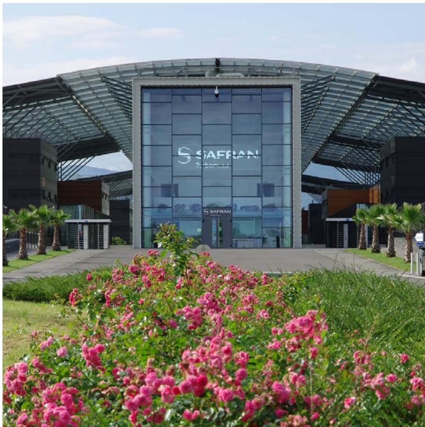
The new Turbomeca Joseph Szydłowski plant
